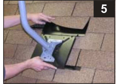
5 Lift upper shingle and slide deck plate under shingle, seat deck plate over base plate
