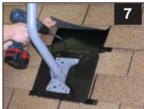
7 Lift shingle, install deck plate using trushead screws, use small amount of roof cement under top shingle
