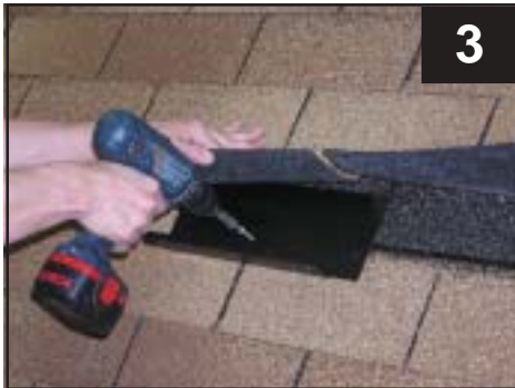
3 Install base plate with trushead screws
