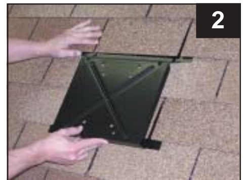
2 Before screwing base plate to roof, align both base & deck plate to assure shingles will fall into place
