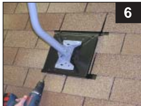
6 Use tek screws to secure deck plate to base plate
